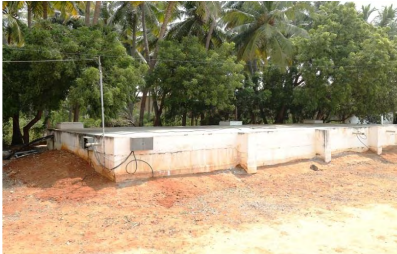
Photo 1: .River intake structure
