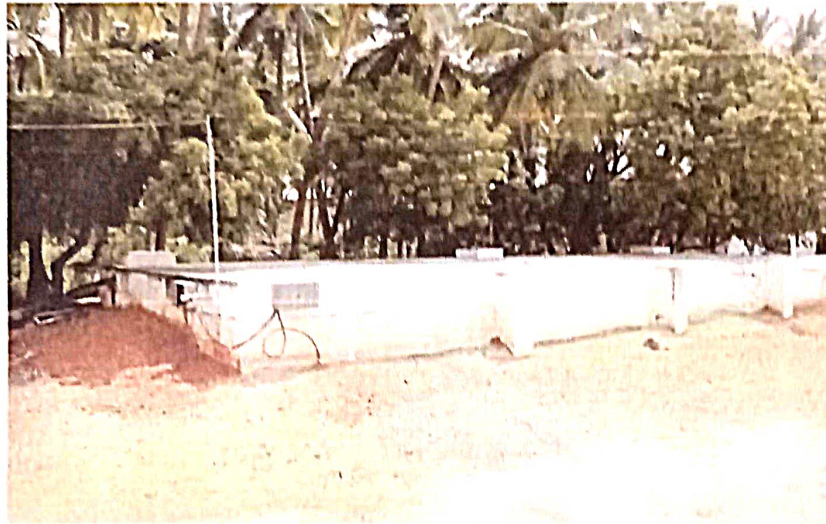
Photo 1: .River intake structure
