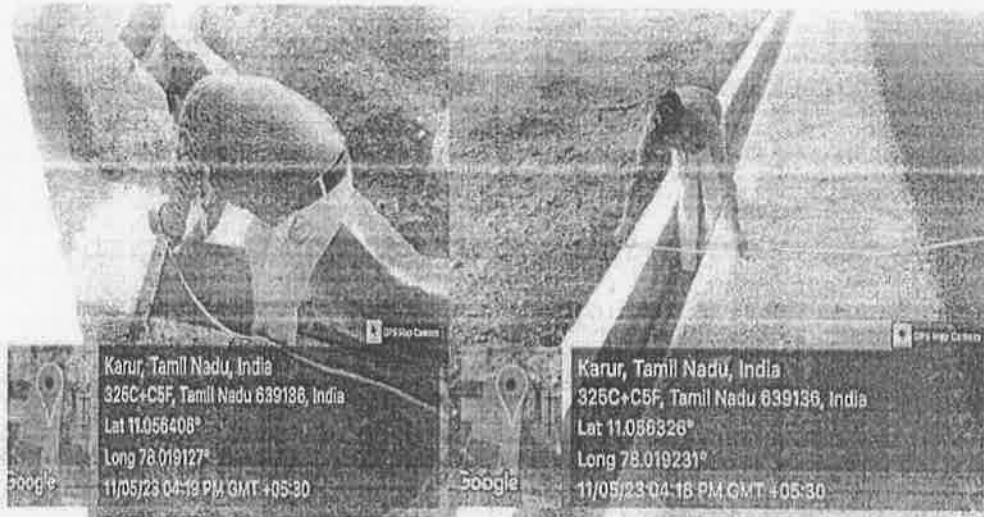
Fig. 3 Storm water drain measurement.
