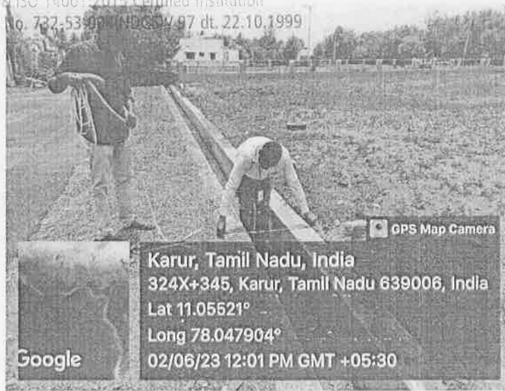
Fig. 3 Storm water drain measurement.
