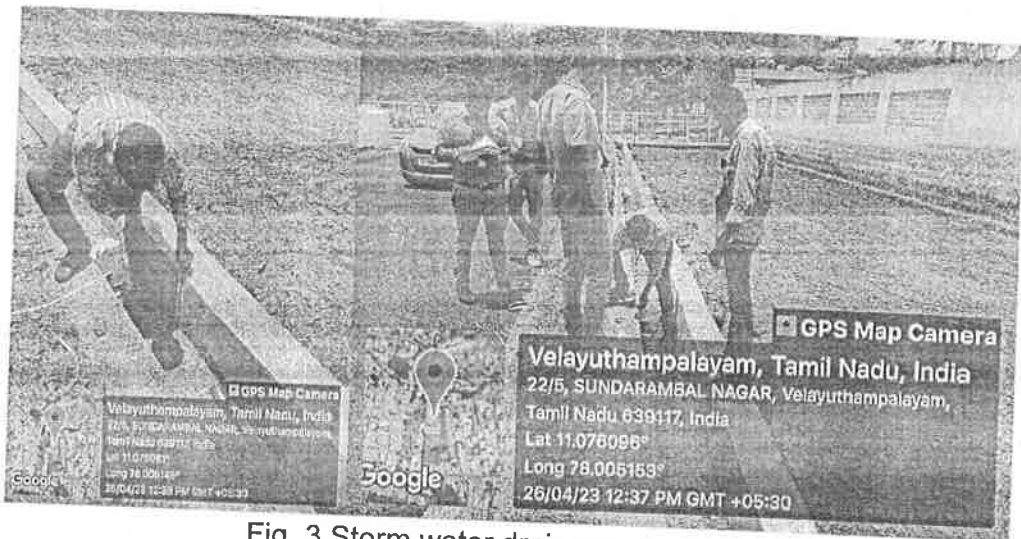
Fig. 3 Storm water drain measurement
