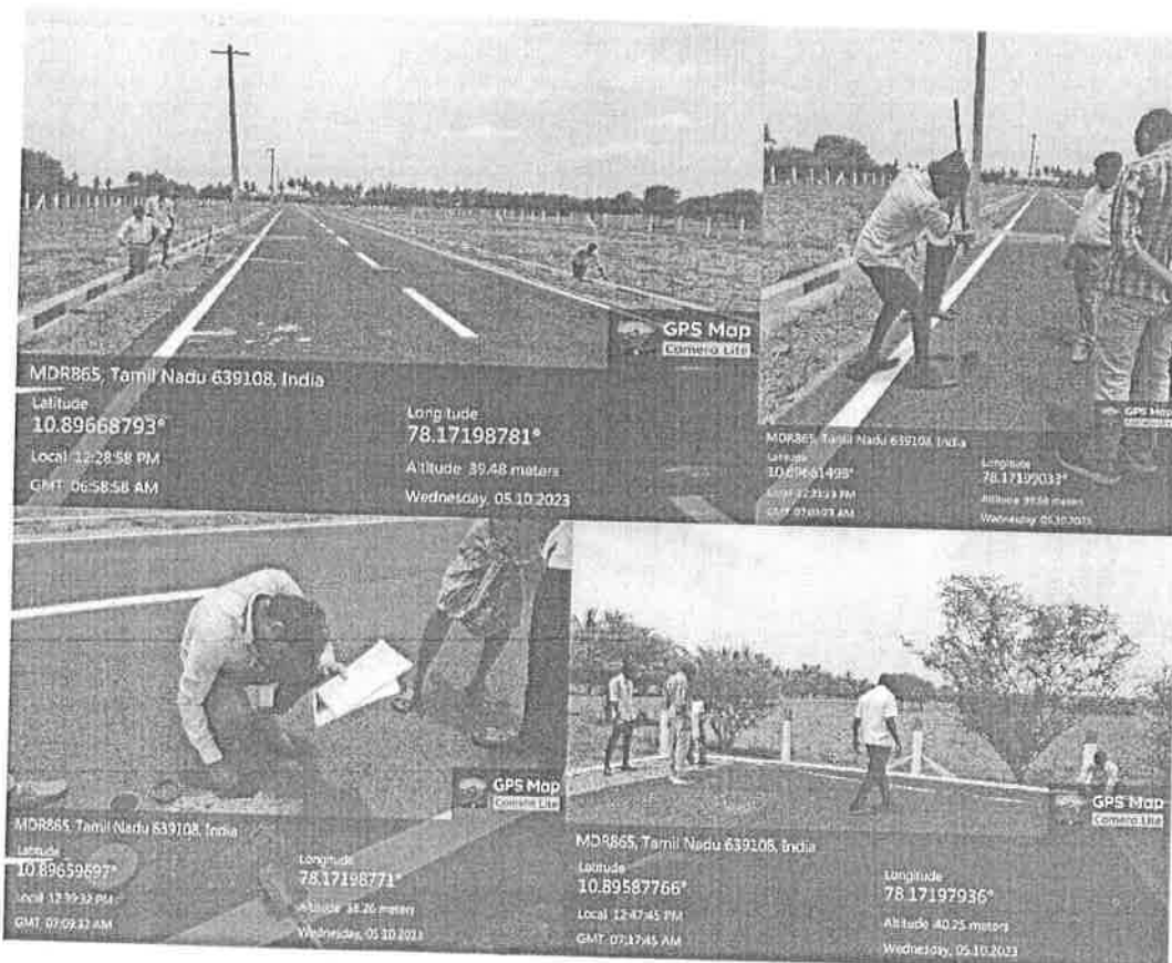
Fig. 2 Road width and cross section measurement
