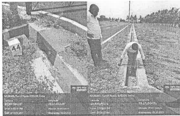
Fig. 3 Storm water drain measurement
