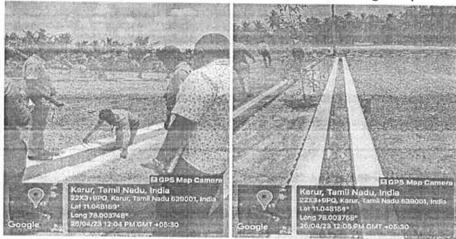
Fig. 3 Storm water drain measurement
