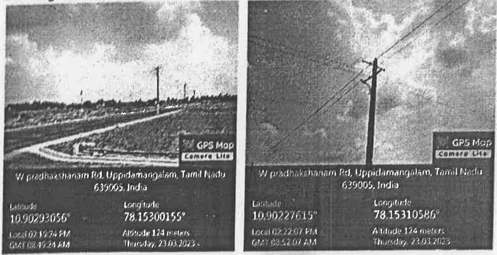
Fig. 7 Provisions of Powerlines & Streetlights
