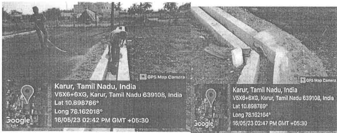
Fig. 3 Storm water drain measurement.
