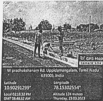
Fig. 3 Storm water drain measurement
