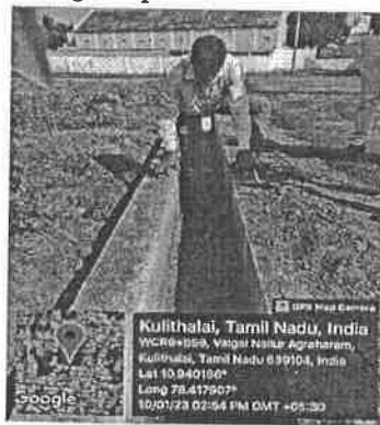
Fig. 3 Storm water drain measurement
