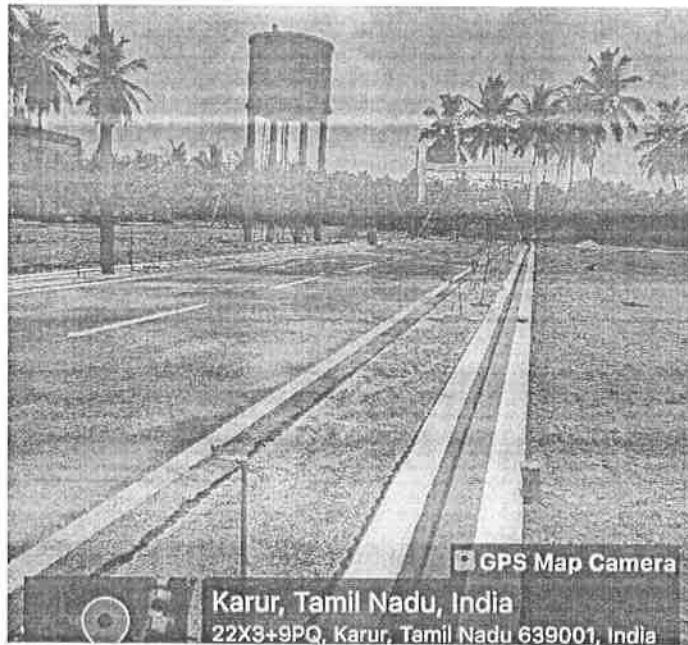
Fig. 5 Provision of Fencing
